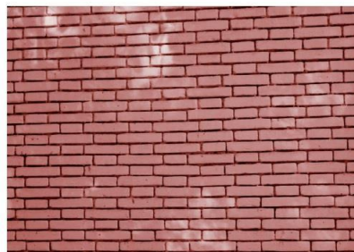
(a) Brick wall
